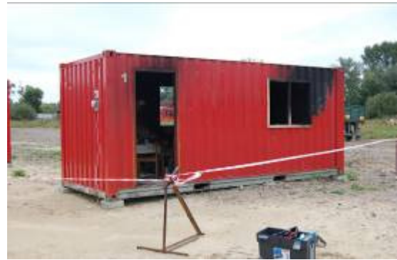
One of the storage containers used for the compartment fires at the training ground in Luboń near Poznań, Poland
